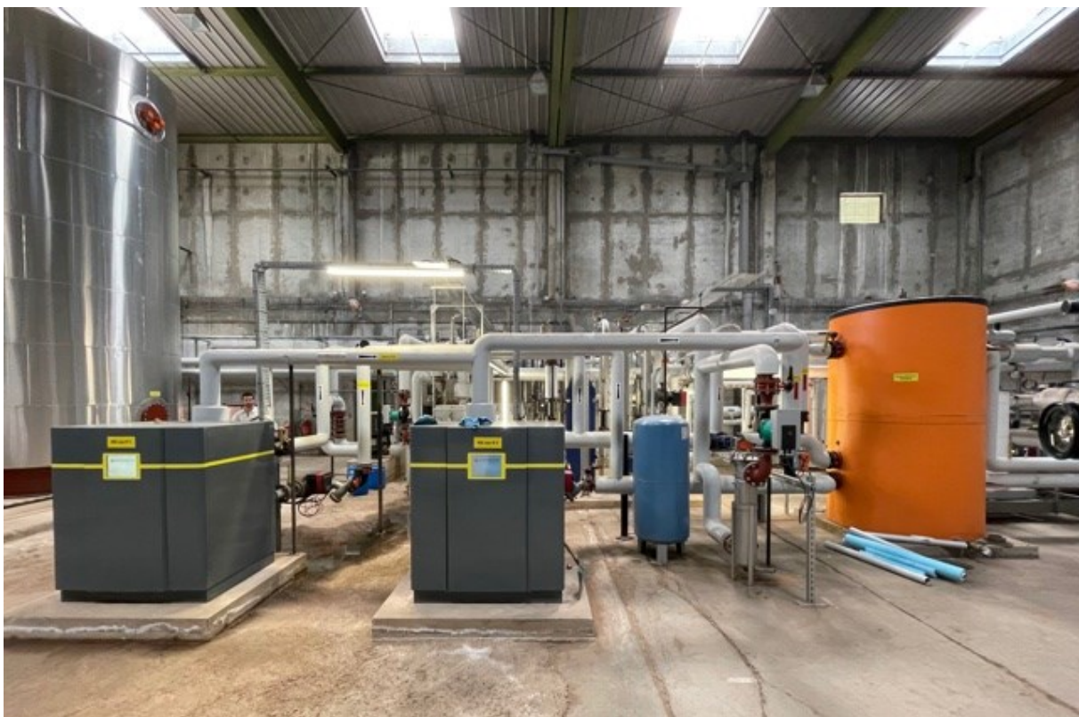
Figure 3.3: View on the main substation as operated today
