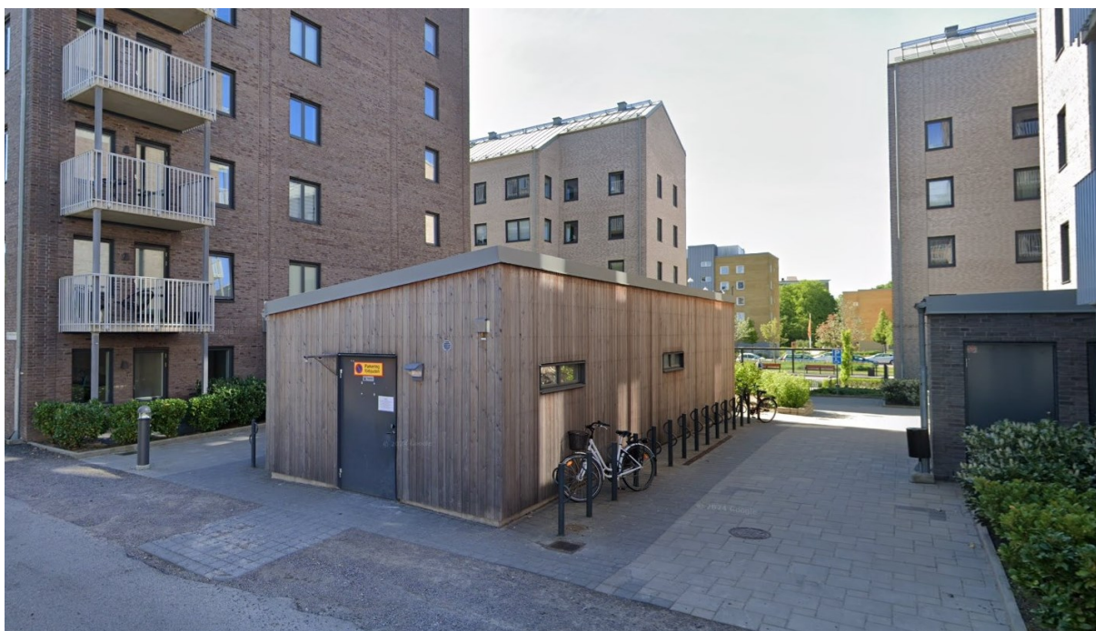
Figure 4.1: The four multifamily homes and the energy centre building
